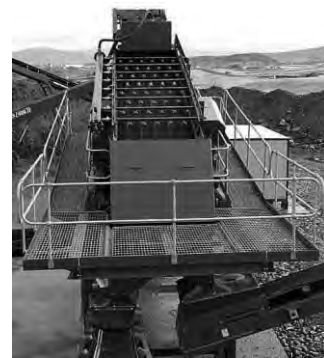
Bolt up structure with galvanized walkways and handrails
